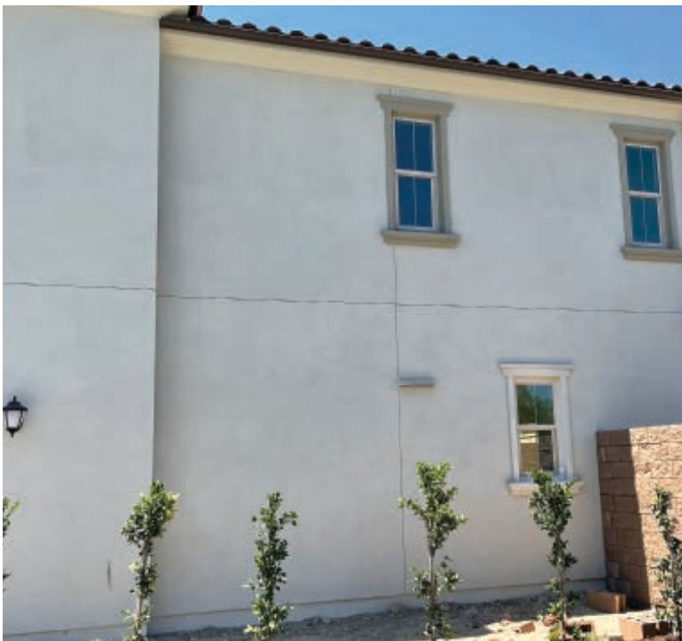
IMAGE 3: STUCCO CONTROL JOINTS
