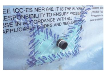
**PROPER INSTALL:** Correctly selected, flashed, and taped housewrap is critical to maintaining an effective weather barrier, especially at penetrations where moisture can easily get through.
