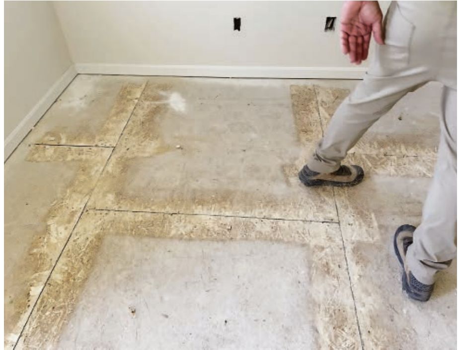
A \frac{1}{8} -inch gap along all panel joints allows for expansion and contraction due to seasonal temperature swings and moisture changes. Without that gap, panels can buckle at the joints and may require sanding to achieve a level floor.
