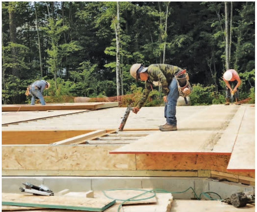
To maintain the glue's integrity, subfloor panels should be installed one at a time and glued to joists before fastening using manufacturer-approved screws or ring-shank nails.
