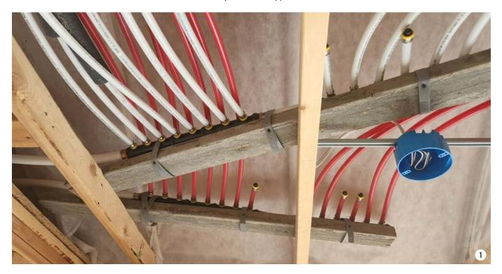
ross-linked polyethylene (PEX) has become the go-to piping for residential water delivery systems, providing a cost-effective, dependable alternative to copper and chlorinated polyvinyl chloride (CPVC). PEX is a popular choice in new construction because it offers flexibility and corrosion resistance, and it's easy to install.
