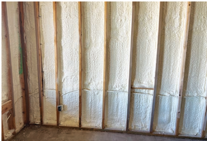
Cavity insulation: Some builders have switched to spray foam insulation (left) due to supply chain issues, which is usually an appropriate swap for fiberglass batts (right) and also provide a greater measure of airtightness and cavity coverage toward a thermally efficient shell.
