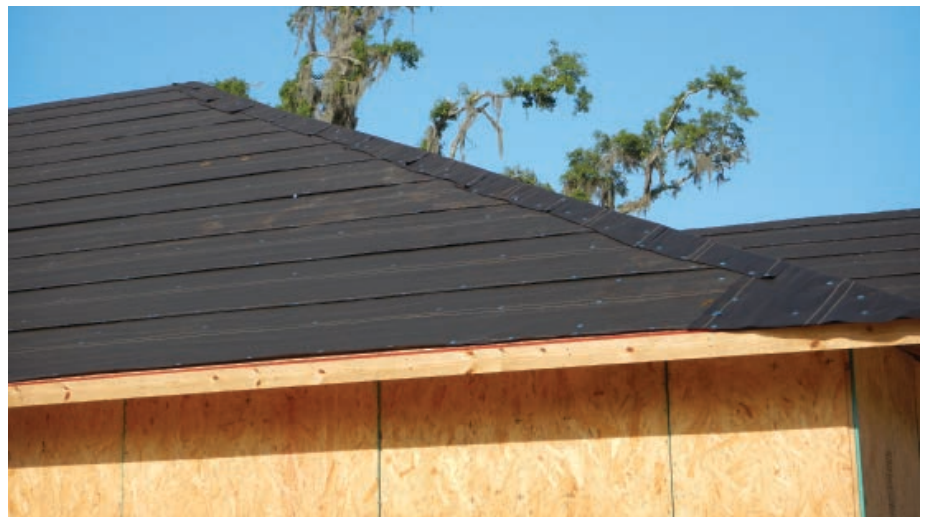
For roof hips and ridges, install underlayment so it overlaps by at least 12 inches.
