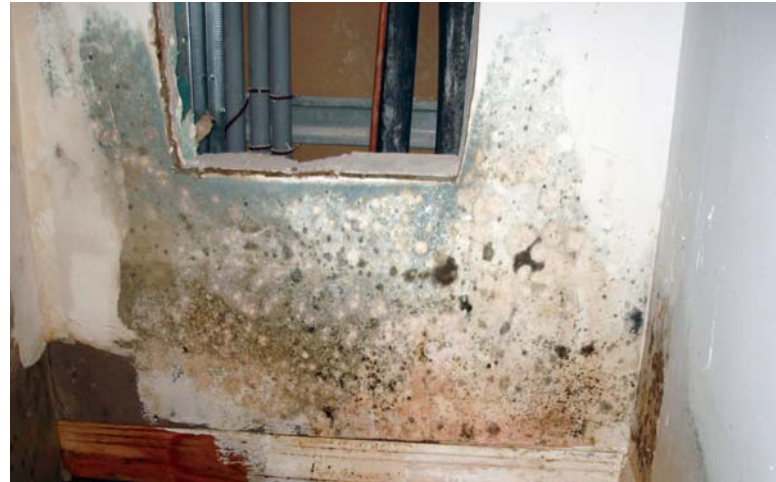
(Above) Mold and other water damage found in most affected units. (Below) New, correctly-sized air conditioning units addressed key remediation issues.
